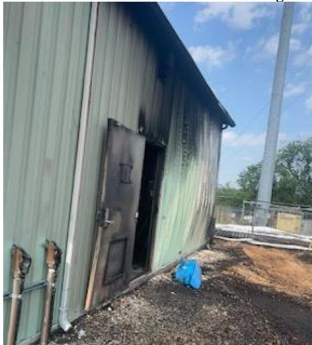
**Photo 7: Gardners Substation Damage**
