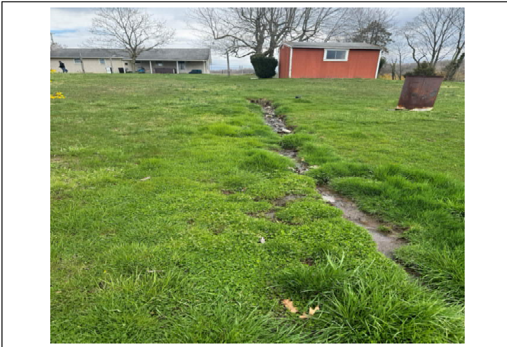
Photo 8: Drainage swale flowing East to West on the back end of the property line. Malfunction of Sewage disposal system (discharging to ground surface)
