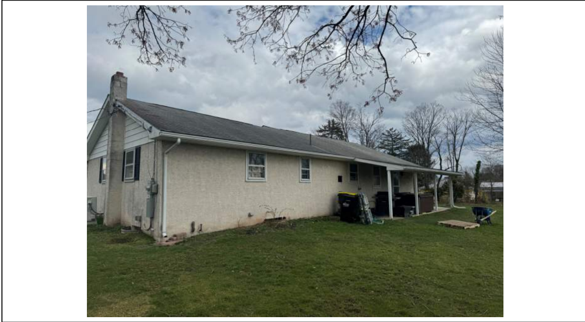
Photo 3: Rear view of the residence (facing East)
