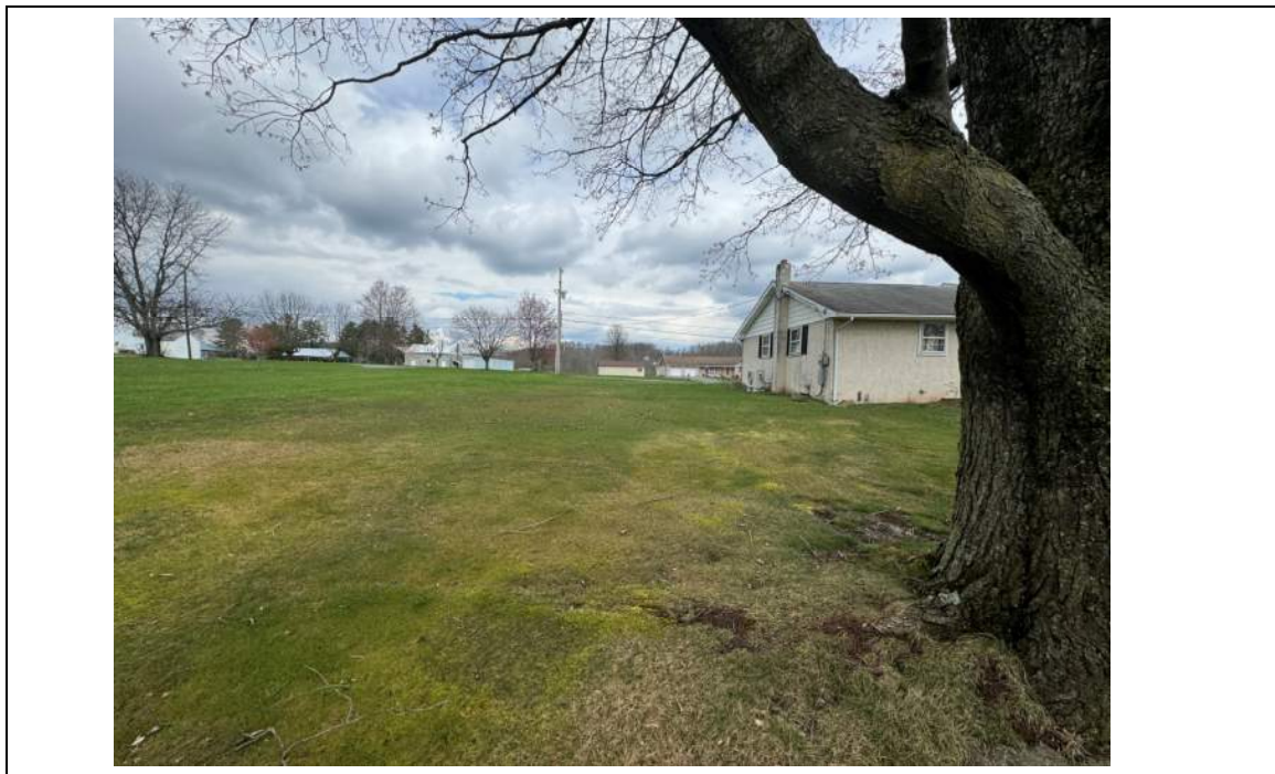
Photo 2: Rear/side view of the residence (facing Northeast)
