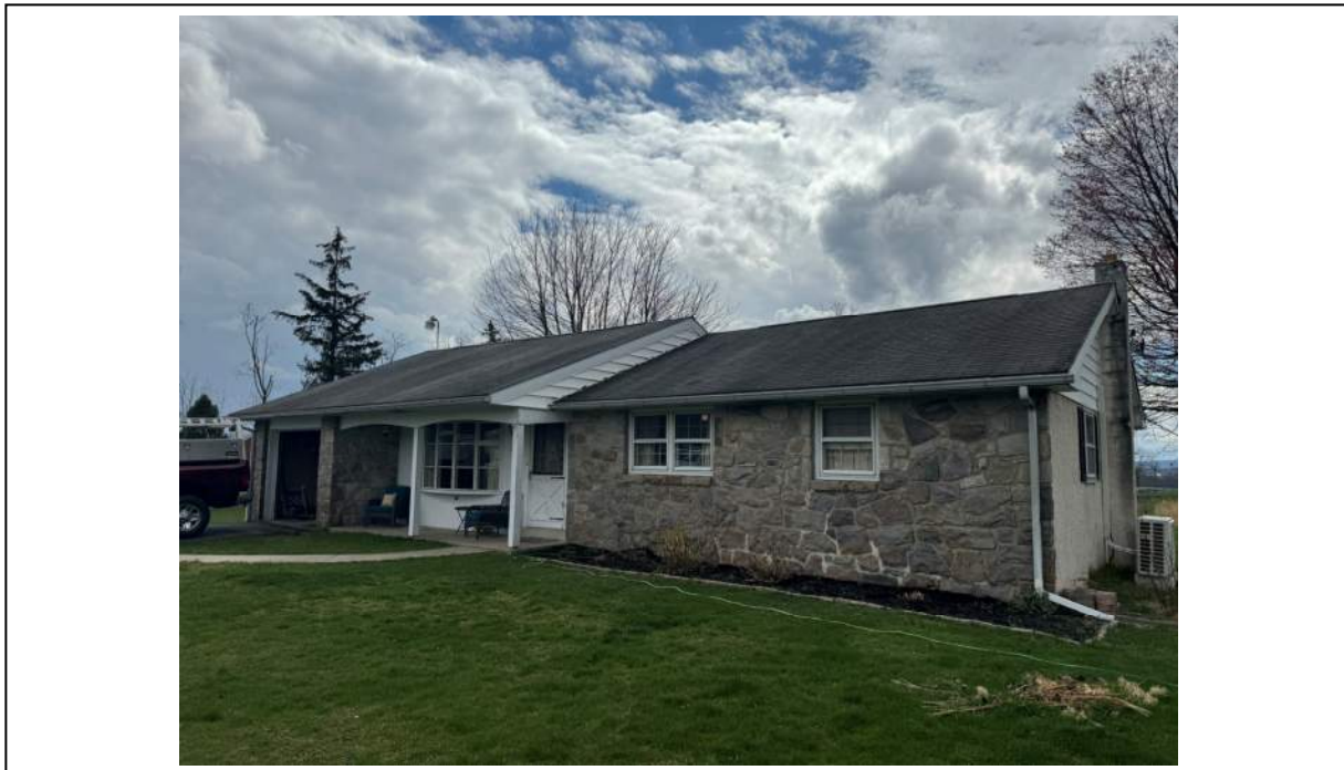
Photo 4: Front view of the residence (South facing)
