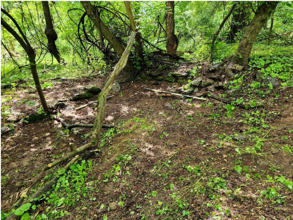
Photograph 16. Site 36YO0500 foundation facing southwest.
