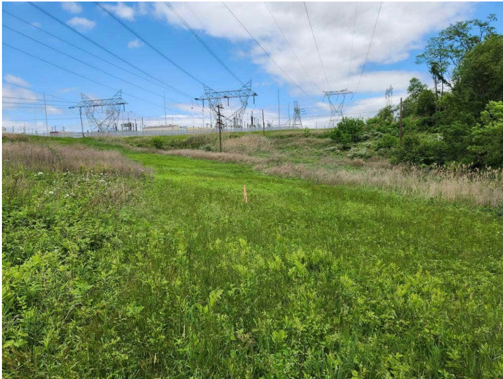
Photograph 11. P174 facing northeast to Peach Bottom North Substation.
