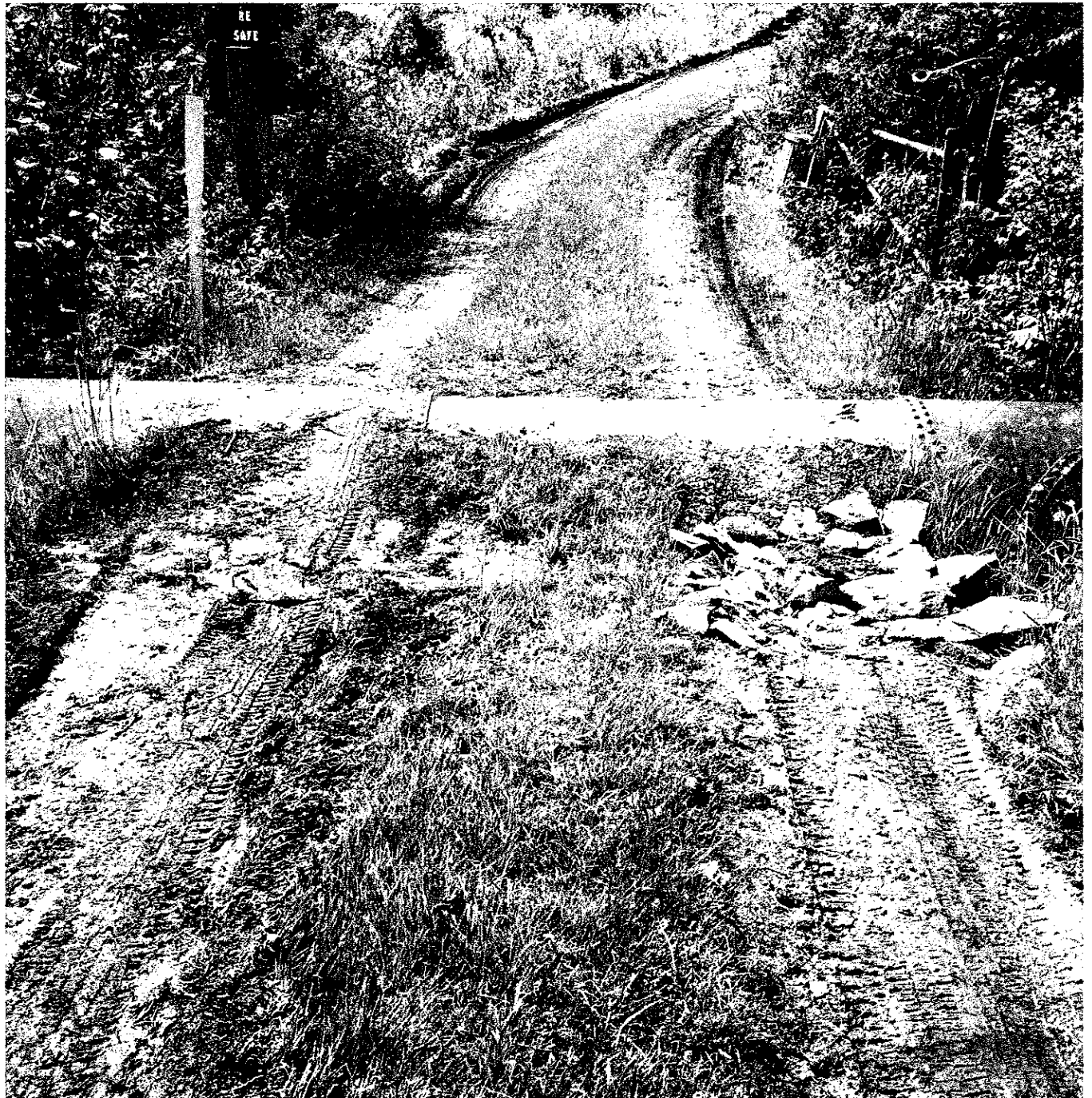
Photo 4 shows another perspective of the collapsed area.
