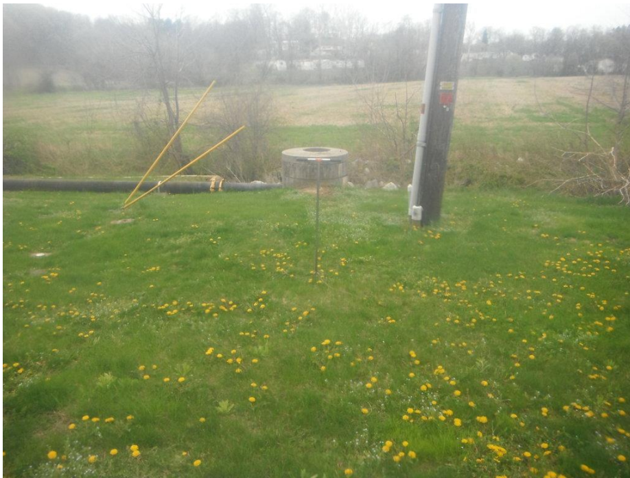
Picture 38 – Looking east at the proposed tie-in location to the existing treatment plant (area of TP-15) (4/14/2025)
