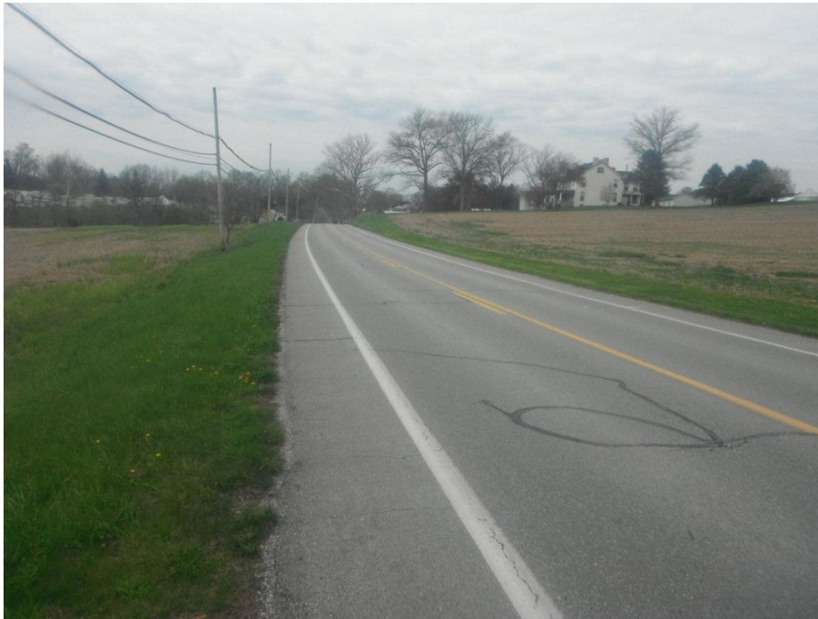
Picture 28 - Looking west along E Prospect Road from the access road to the existing treatment plant (4/14/2025)
