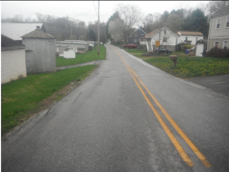
Picture 11 – Looking north along 1 st Street toward the Furnace Road intersection (4/14/2025)
