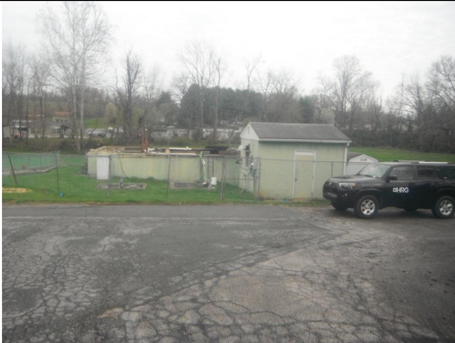
Picture 1 - Looking north at the existing mobile home park treatment facility in the southwestern portion of the Project Area (4/14/2025)
