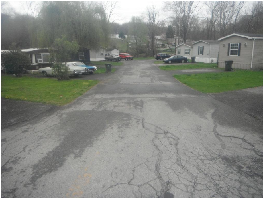
Picture 12 – Looking south along 1 st Street from the Furnace Road intersection (4/14/2025)
