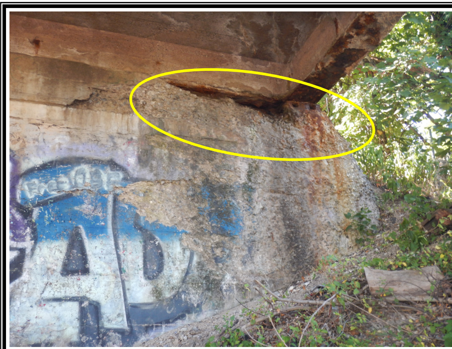
FAR ABUTMENT BRIDGE SEAT Right End
