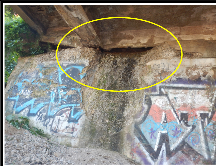
FAR ABUTMENT BRIDGE SEAT Left End
