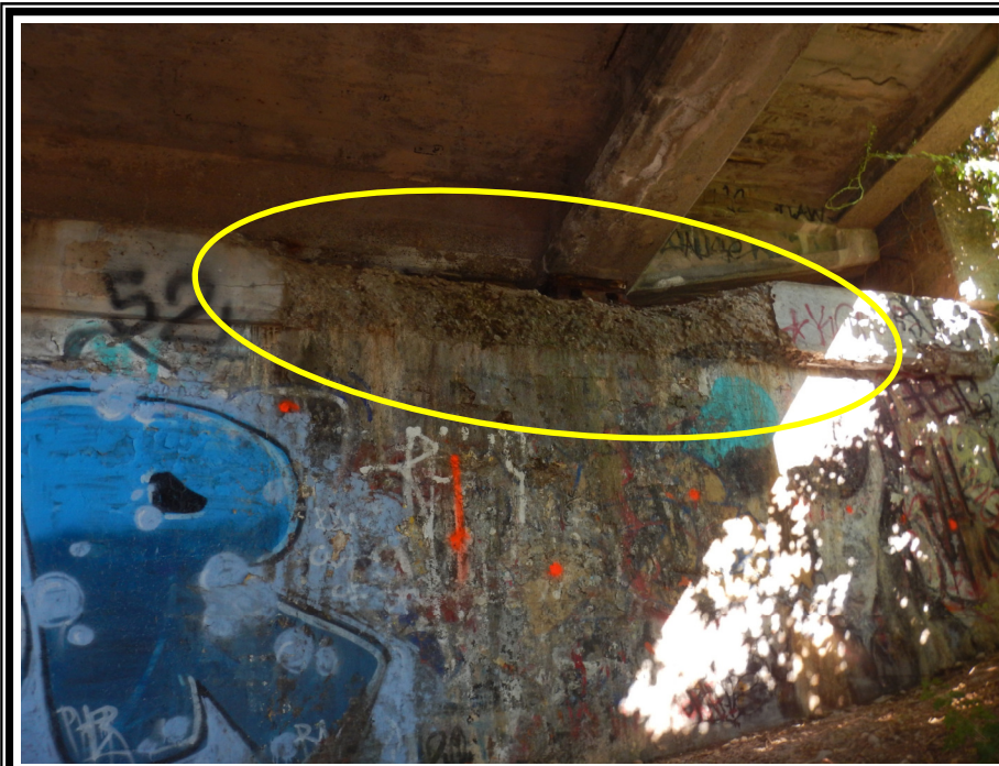
NEAR ABUTMENT BRIDGE SEAT Left End
