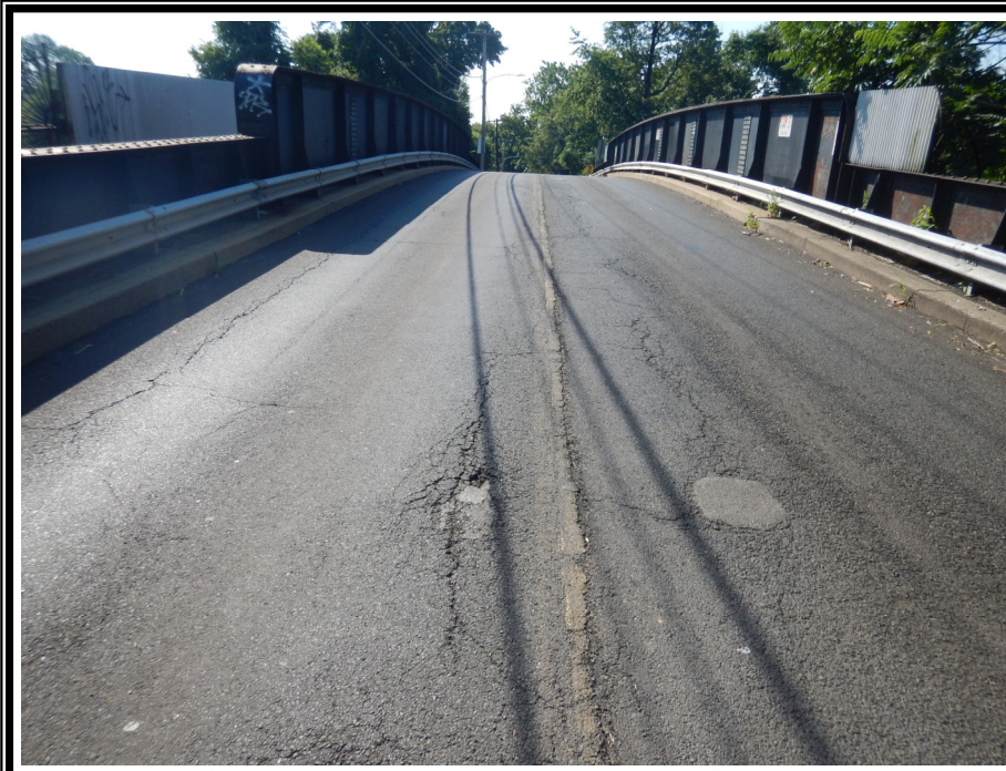
GENERAL VIEW OF THE WEARING SURFACE
