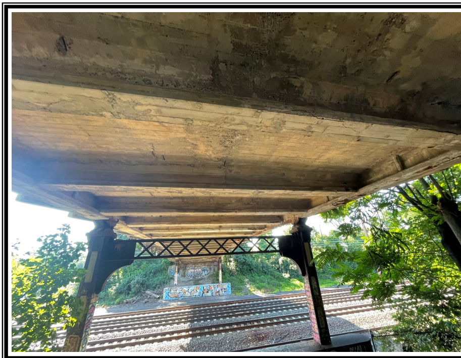
SPAN 1, GENERAL VIEW OF THE UNDERSIDE Looking Ahead
