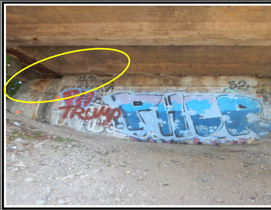
NEAR ABUTMENT BRIDGE SEAT Right End
