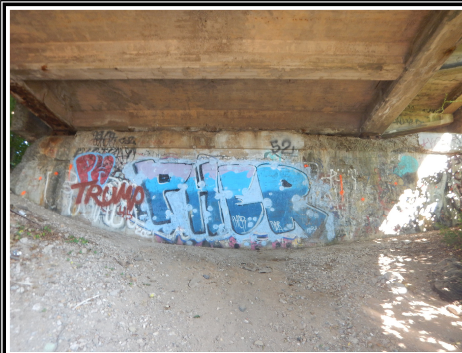
NEAR ABUTMENT West
