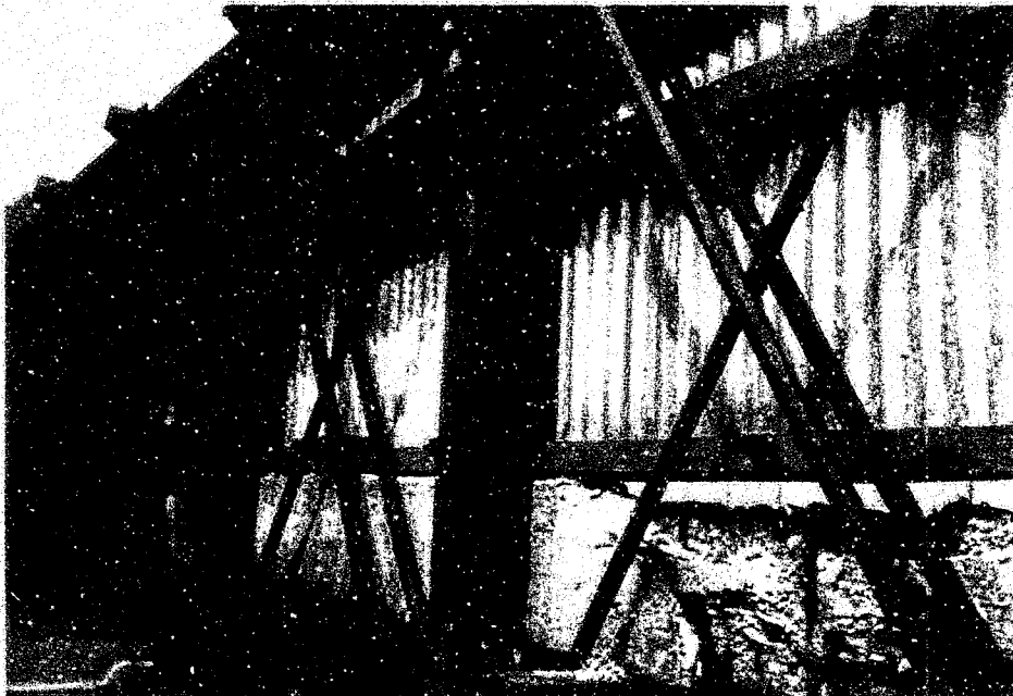
2. West truss, north end, disconnected arch ring and spalled concrete.
