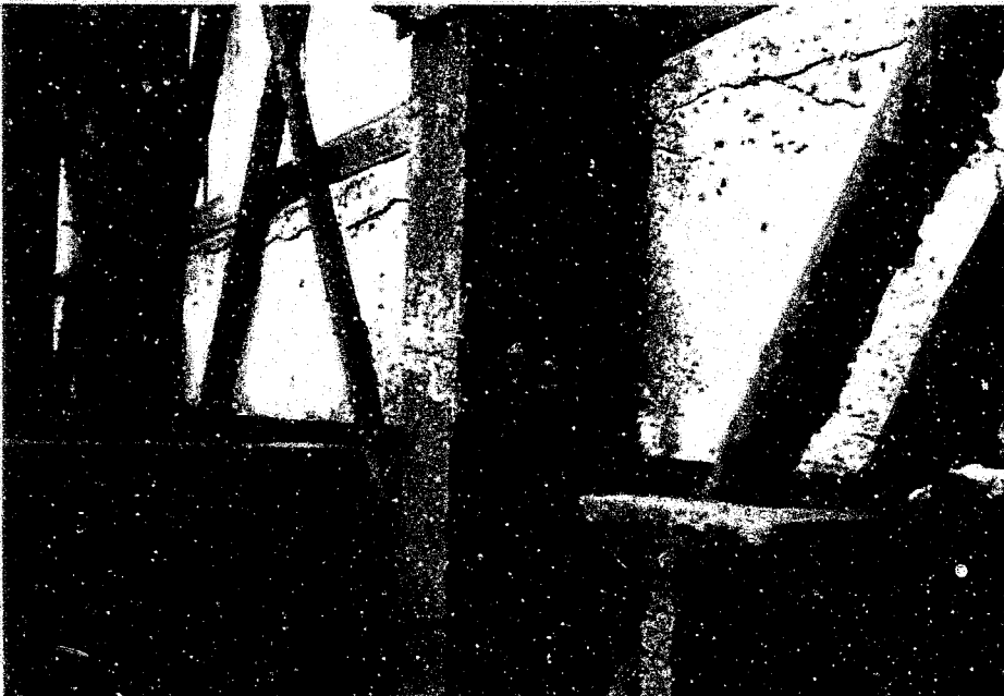
8. Closer view of crack in 5th vertical.
