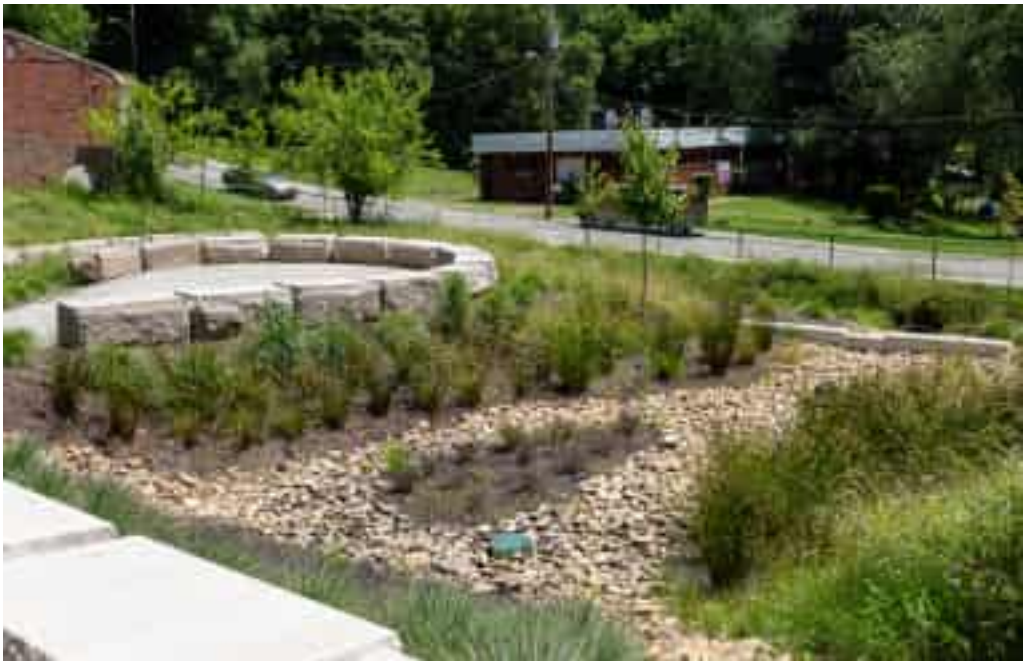
Hillcrest Green Stormwater Infrastructure, Pittsburgh
