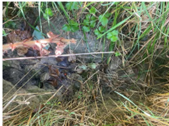
SPA-JRW-003 Facing W (09/19/24)
