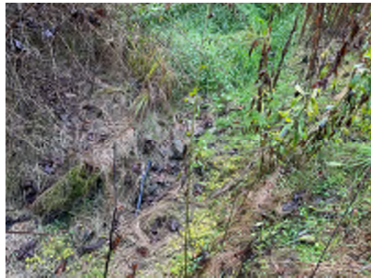
SPA-JRW-004 Facing N-NE (09/19/24)
