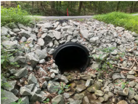
Stream SPA-JGG-001 Facing E-NE (07/31/25)
