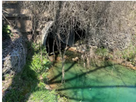
Stream SPA-BJY-002 Facing W-SW (04/23/25)
