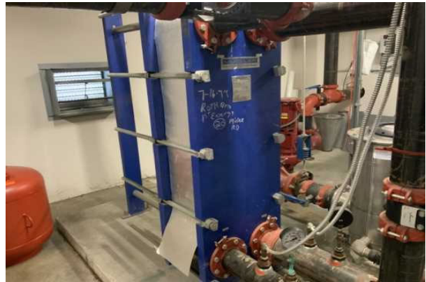
28 HEAT EXCHANGER, PLATE AN FRAME
