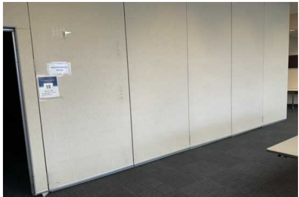
42 INTERIOR WALL CONSTRUCTION, MOVABLE PARTITIONS, FABRIC
