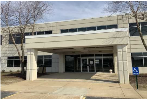
3 RIGHT SIDE ENTRANCE
