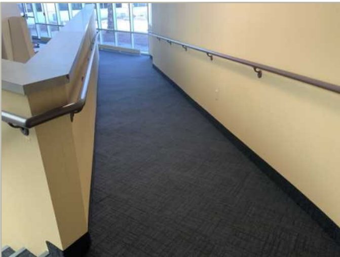
Access ramp to the Atrium
