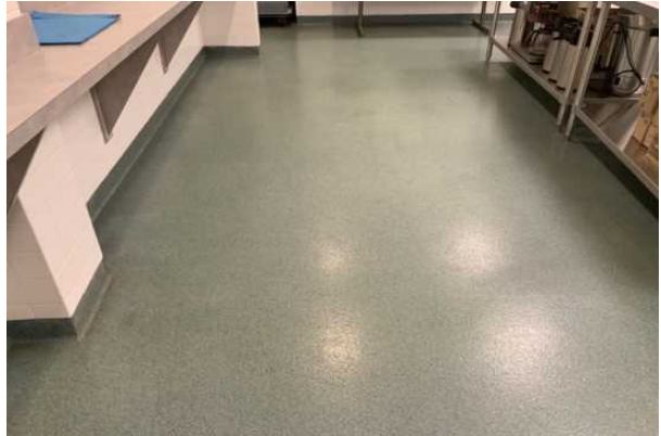
38 FLOORING, TERRAZZO, REPLACE
