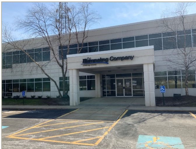
Main accessible entrance and primary path of travel
