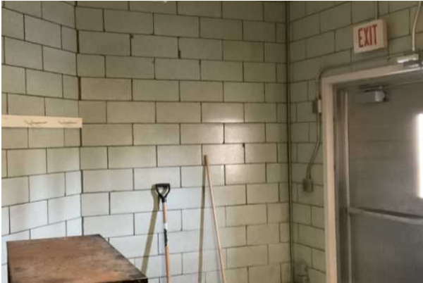
45 WALL FINISHES, QUARRY TILE
