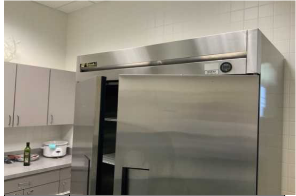
26 FOODSERVICE EQUIPMENT, REFRIGERATOR
