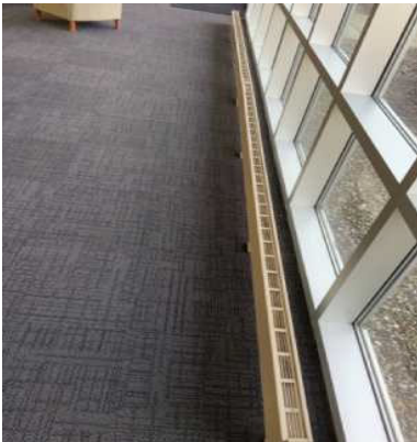
39 BASEBOARD HEATER, ELECTRIC, 4 LF, 1 KW, REPLACE
