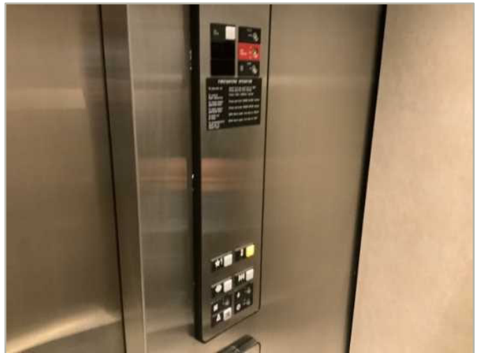
Elevator cab interior
