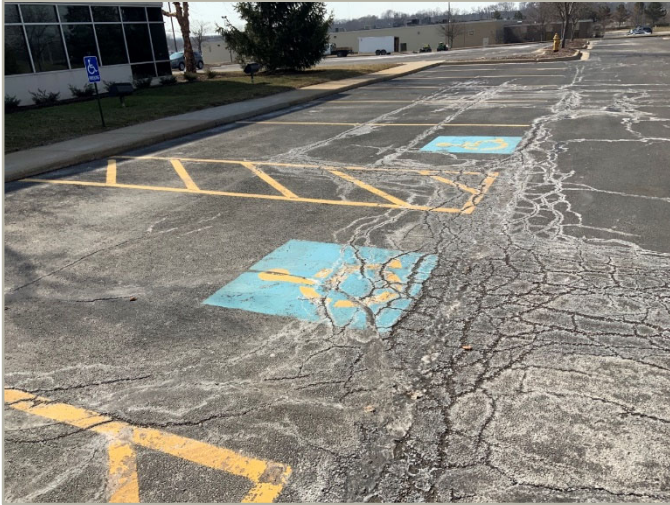
Overview of accessible parking area
