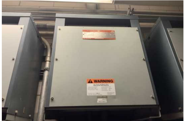
14 SECONDARY TRANSFORMER
