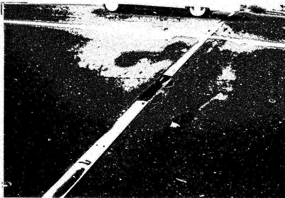
North End Expansion Joint Northbound Side
