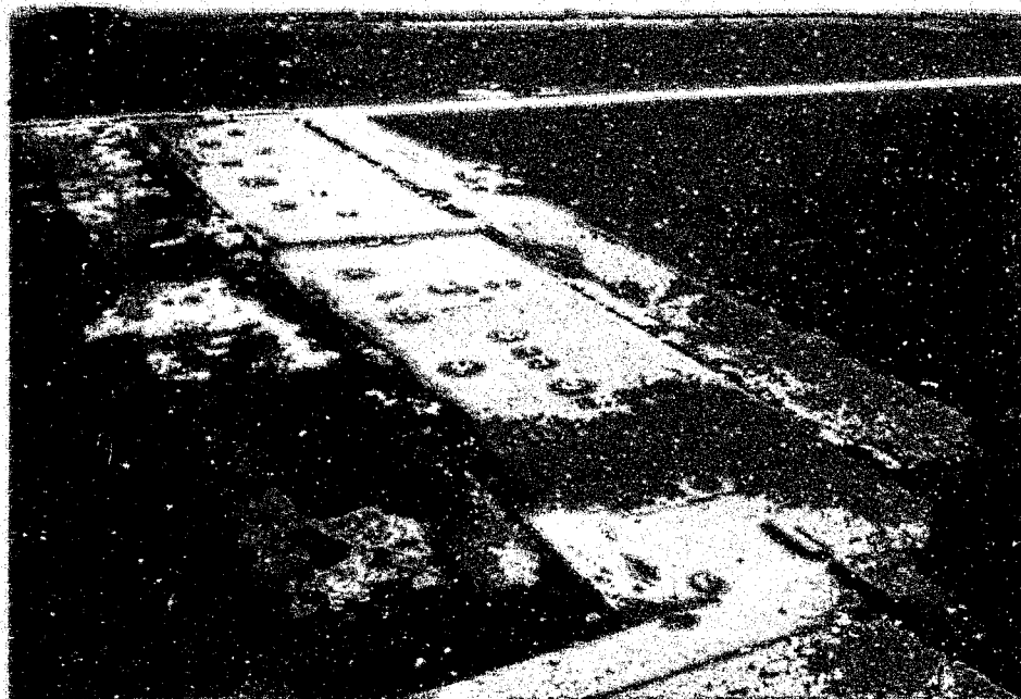
South End Expansion Joint Northbound Side
