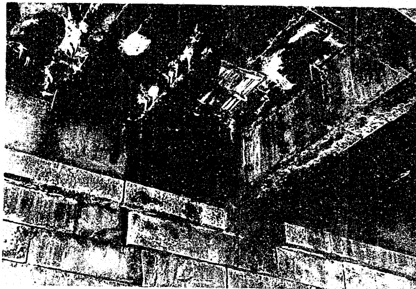
10. Under side of deck at east side of Pier #1, showing deterioration of slab and cracks in stone masonry.
