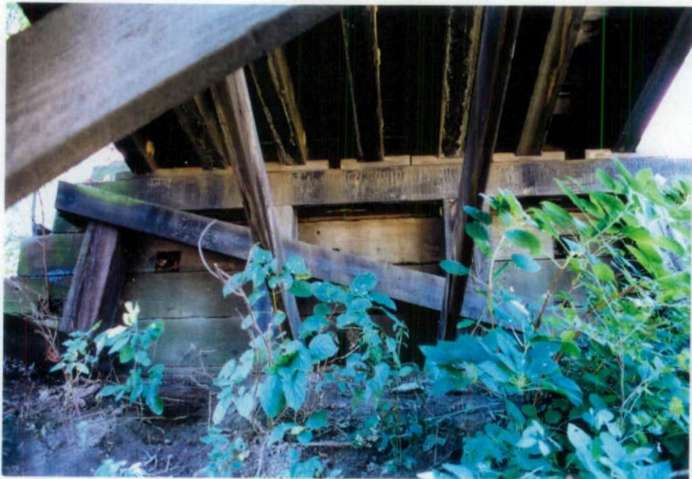
GENERAL VIEW OF SOUTH ABUTMENT
