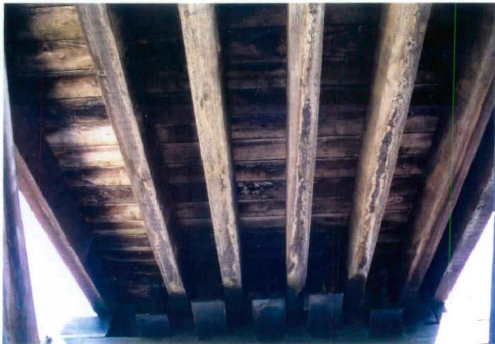
GENERAL VIEW OF TIMBER STRINGER SPAN
