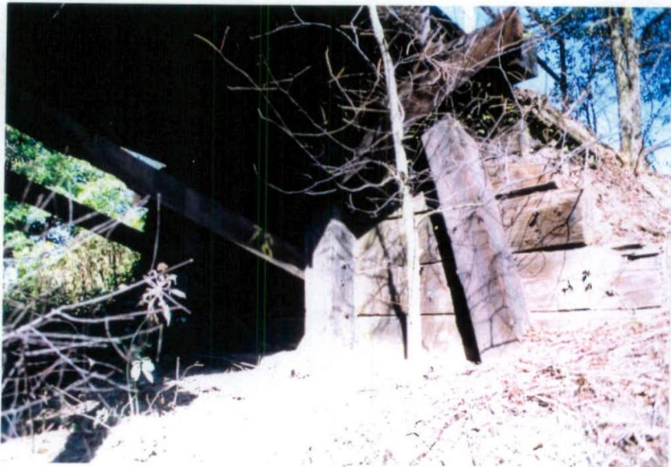
GENERAL VIEW OF NORTH ABUTMENT
