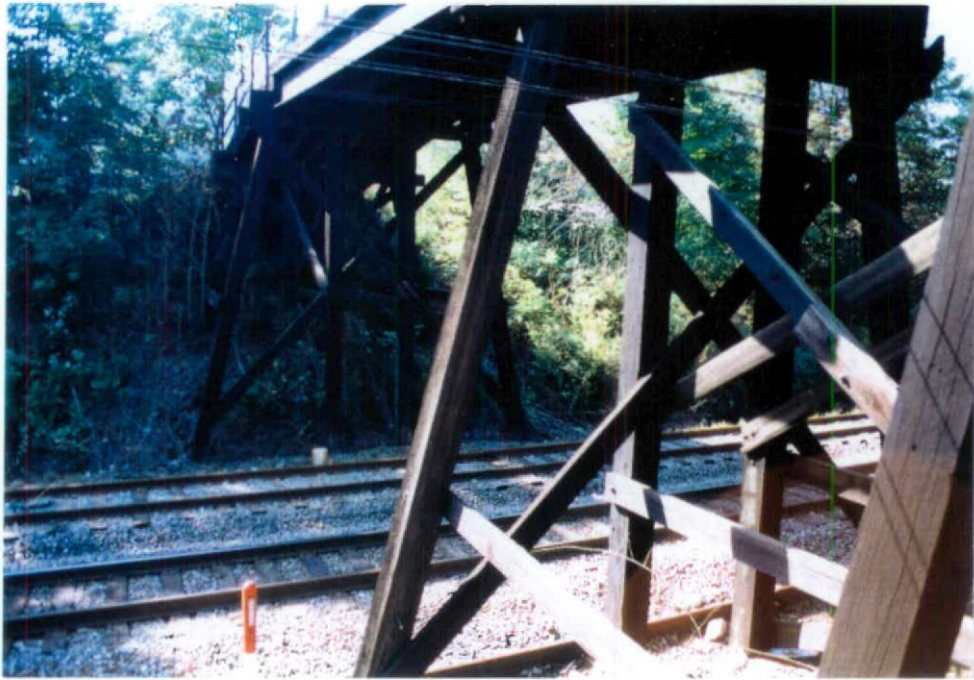
5. GENERAL VIEW OF STEEL STRINGER SPAN 3 AND TIMBER BENT NOS. 2 AND 3
