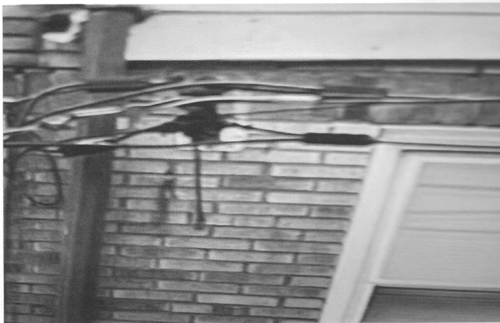
Photo #5 Taken 04/26/2026 - "Visible impression of the original bracket above the current bracket. The outline is clean and sharply defined, indicating the original bracket has recently detached having causing severe Wall Damage prior to dislodging.
