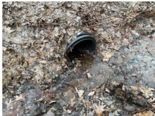
Stream SPA-REW-004 Inflow Culvert Facing North (02/05/25)
