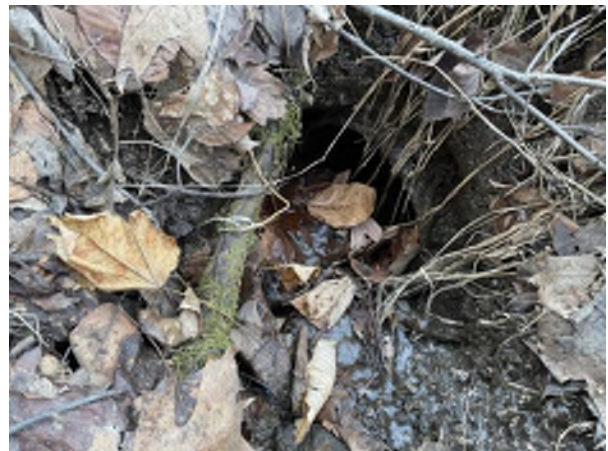
Stream SPA-REW-002 Inflow Culvert Facing North (02/05/25)
