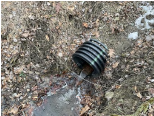
Stream SPA-REW-004 Outflow Culvert Facing South Facing (02/05/25)
