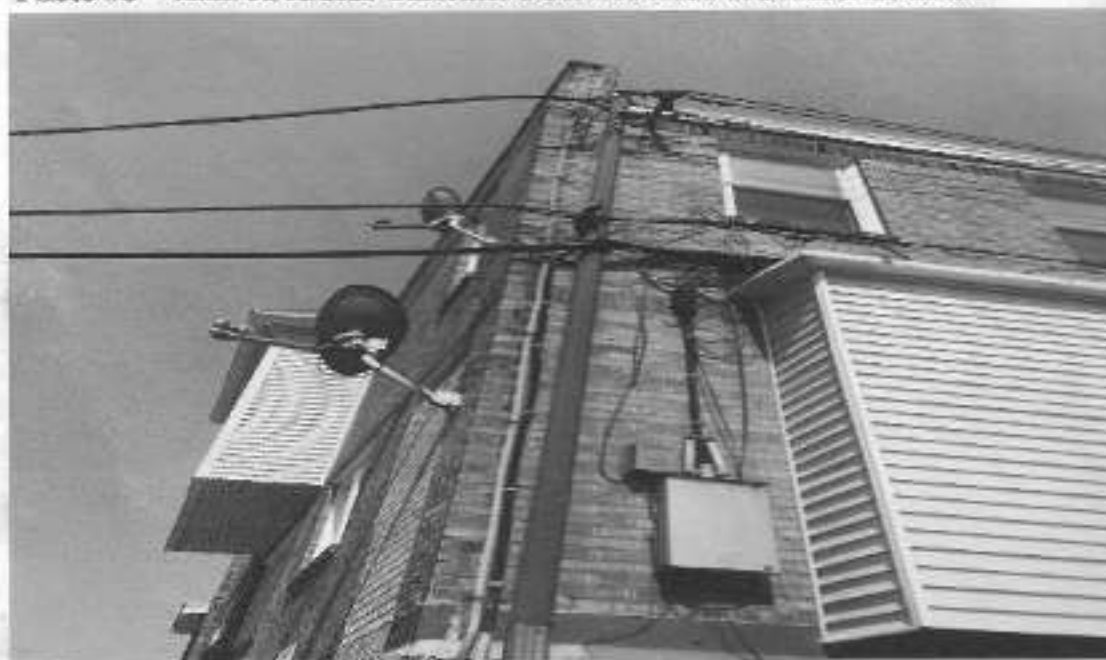
Photo #8 – Taken 06/01/2023 Customer's Service Head & Bracket Location
