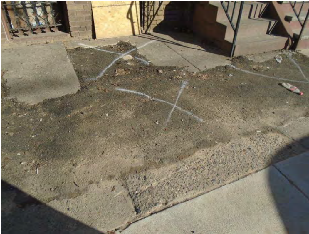
Photograph #40: Sidewalk area in the front of 815 Jackson Street where plumber worked.
