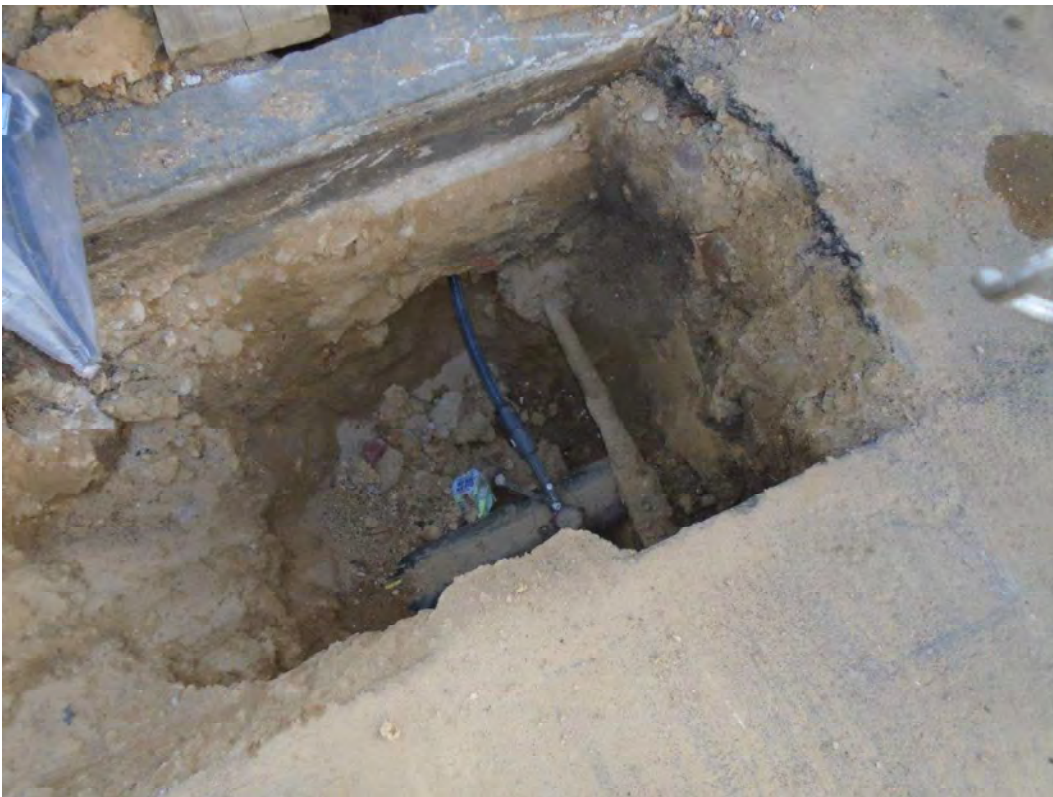
Photograph #4: Gas pipe lateral to 818 Jackson Street.
