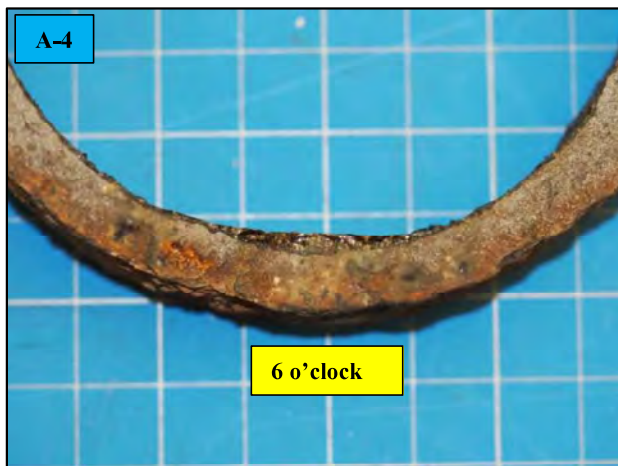
Photo No. 32 (W-6491-E-086.JPG)
