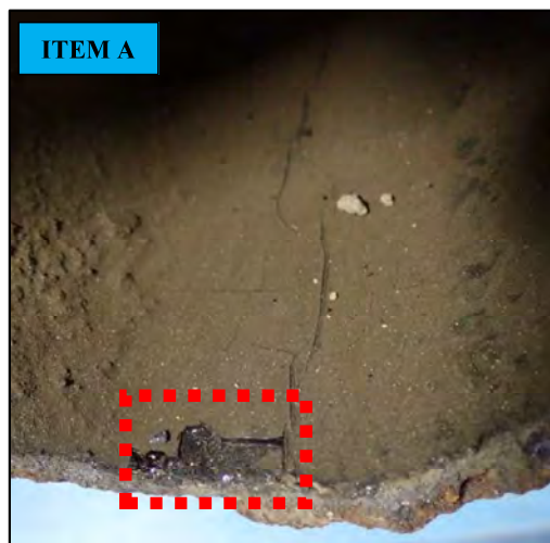
Photo No. 11 (W-6491-D-162.JPG)
