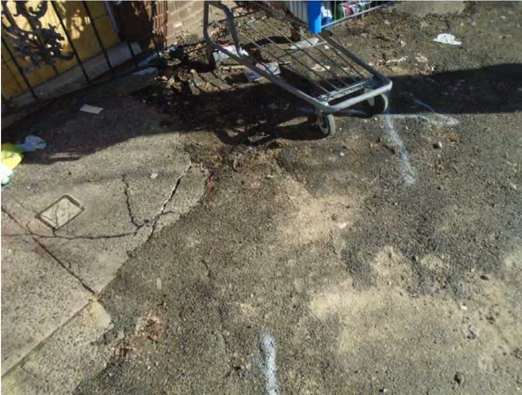
Photograph #37: Sidewalk area in the front of 815 Jackson Street where plumber worked.
