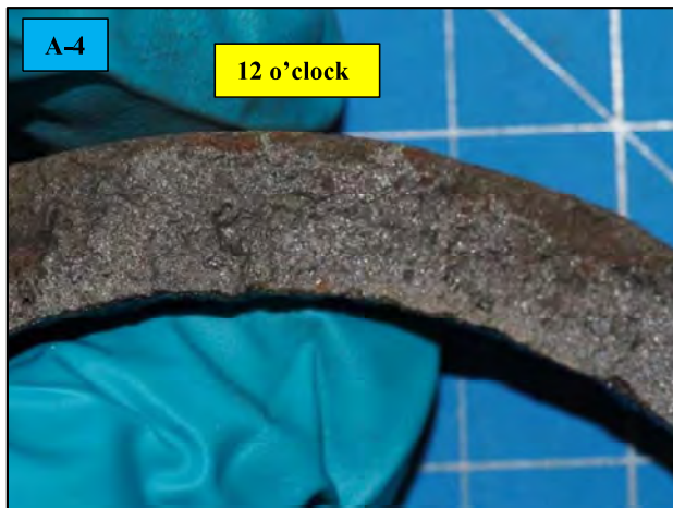
Photo No. 30 (W-6491-E-096.JPG)
