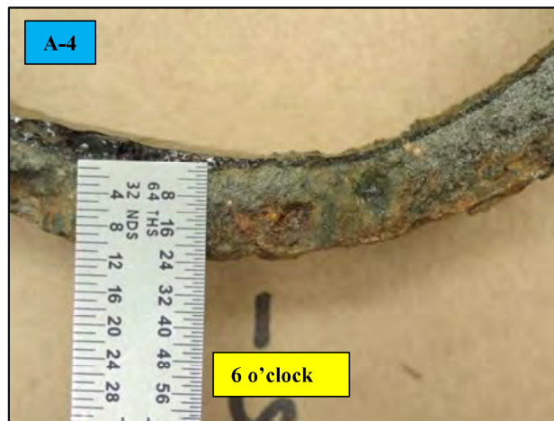
Photo No. 34 (W-6491-D-250.JPG)
