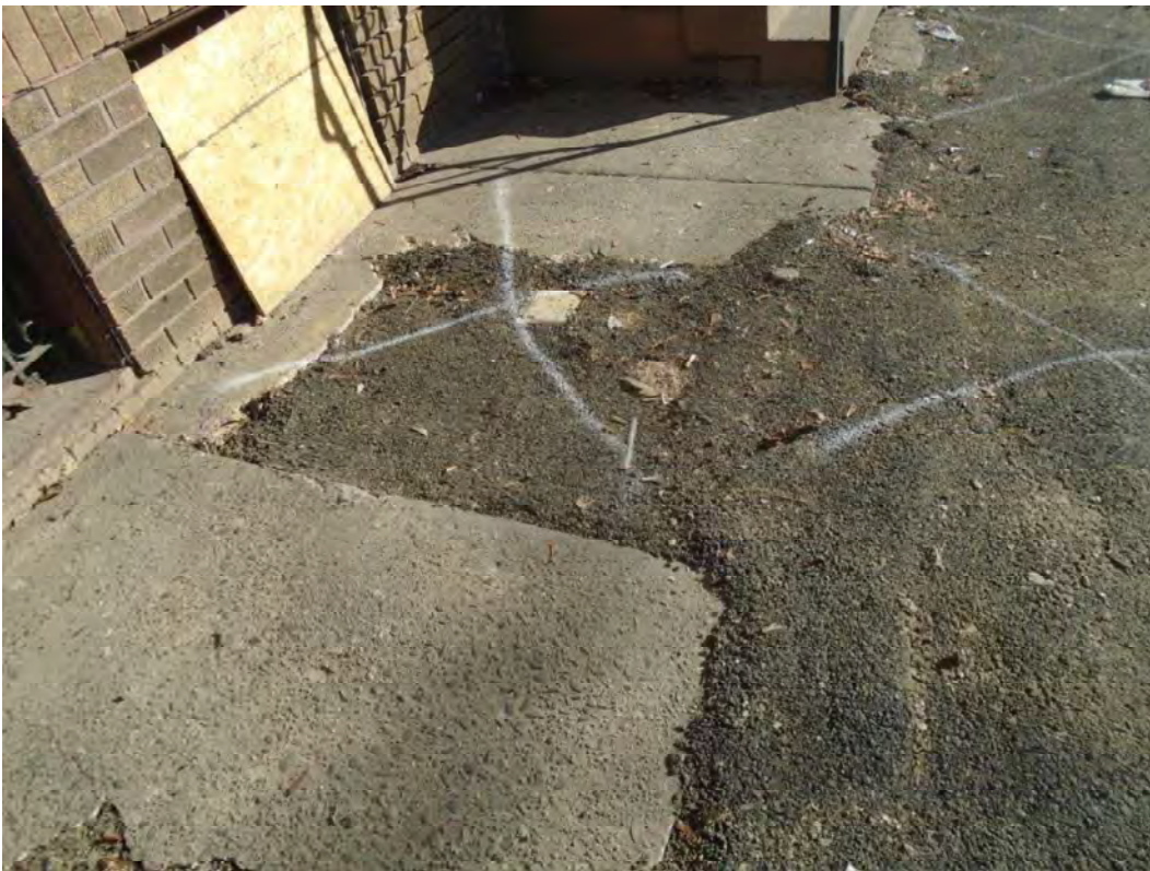
Photograph #38: Sidewalk area in the front of 815 Jackson Street where plumber worked.
