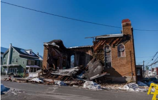
Damage seen at a former synagogue at the corner of West Mahanoy and South Catawissa streets in Mahanoy City on Feb. 13, 2026. The building partially collapsed the night of Feb. 12. FILE
